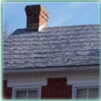
The original pressed tin shingles, a representation of the preferences and technologies of time, have been retained.
