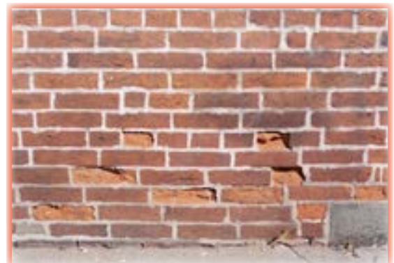
This brick wall was incorrectly repointed, causing the brick faces to fracture and crumble.
