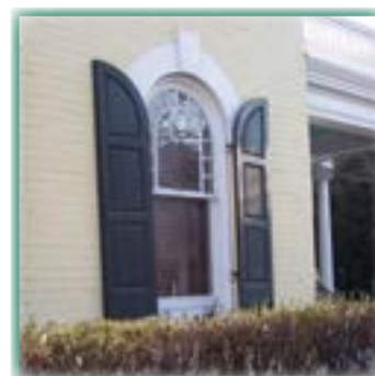
These shutters are functional and fit the size and shape of the window opening.
