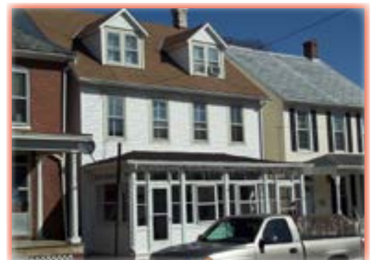
The porch on the right was inappropriately enclosed using permanent materials that change the character of the porch.
