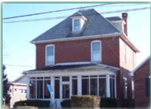
The screens on the porch to the left were installed behind the porch columns, preserving the open character of the porch.
