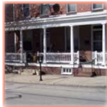
The porch steps on the left have inappropriately been replaced with concrete.
