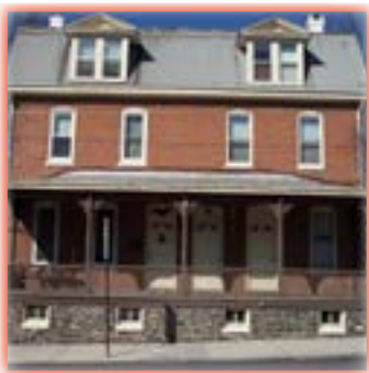
The door on the far right was converted from a window opening. This conversion has interrupted the rhythm of the façade, creating an uneven appearance.
