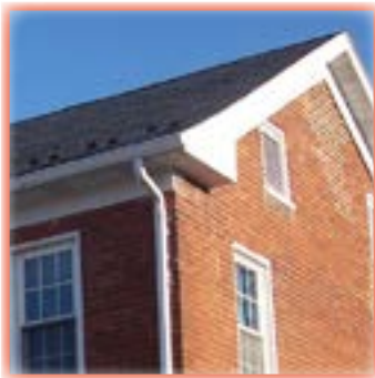
The cornice has been boxed in with modern materials, altering the architectural character of this house.
