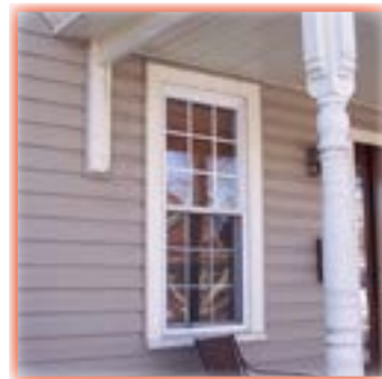
These modern replacement windows do not retain the visual qualities of true divided-lite windows.
