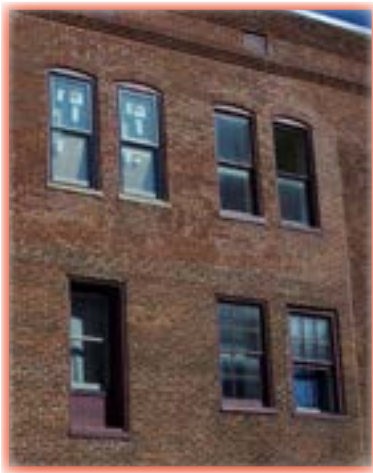
The windows in this building are being replaced with modern windows. Though they match the arrangement of some of the originals, they are not an appropriate substitute for wooden true divided-lite windows.
