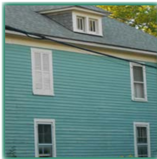
This window is no longer used but the integrity of the façade has been maintained by using shutters to close the opening.
