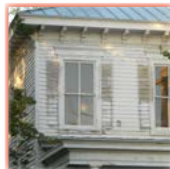
The shutters on this building have been removed.
