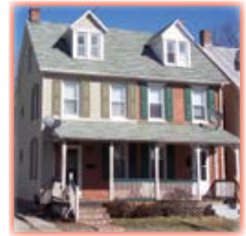
Half of this house has been inappropriately covered with vinyl siding.
