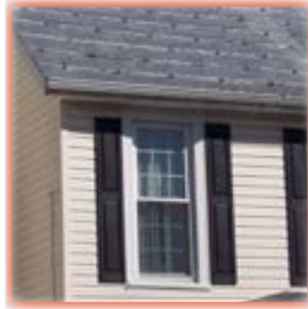
These shutters are too small for the window opening and they are mounted directly onto the wall.
