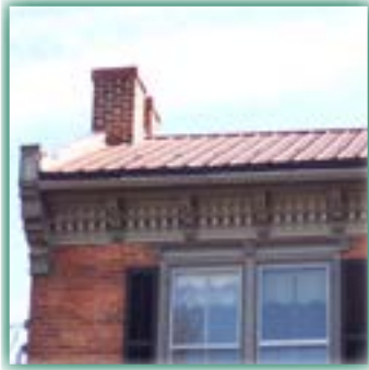
This elaborate bracketed cornice has been retained, preserving the integrity of this Italianate house.
