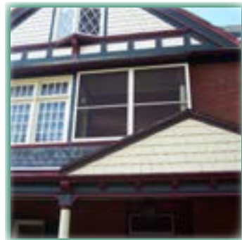
The screens on this small porch appear to be removable. When they are not being used the porch can be returned to its original state.
