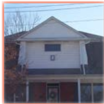
The window opening on this dormer has been reduced, changing the character of the façade.
