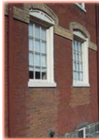
These windows were inappropriately resized.
