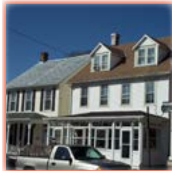
The dormer windows on this building are most likely a later addition and are not compatible with the rest of the houses on the street.
