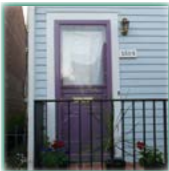
This storm door does not cover the original door and has been painted to match.
